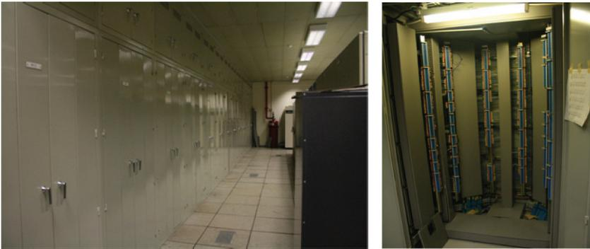
Fig. 1. I/O Cabinets and wiring cabinet.
