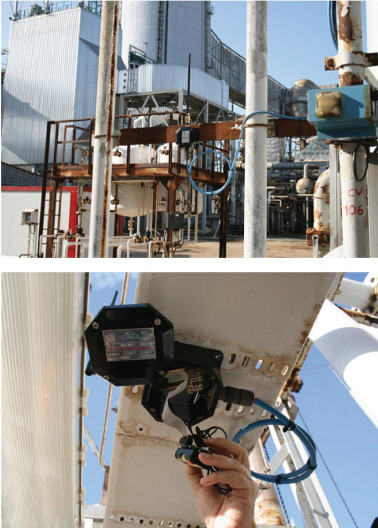
Fig. 12. Sensor nodes deployed in the refinery.
